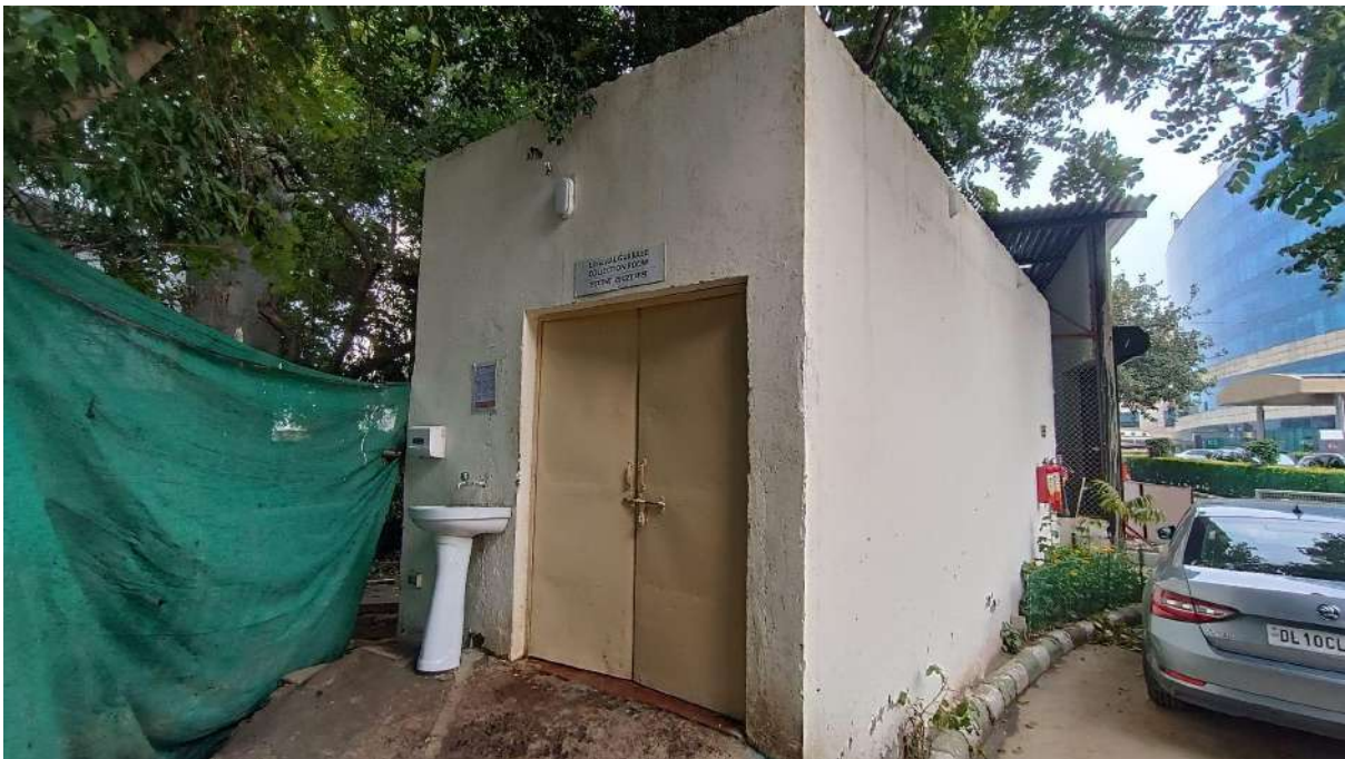
Photograph :- Municipal Solid-Waste Storage Area
