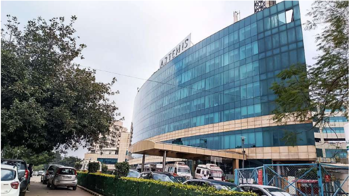
Photograph :- Operational Building
