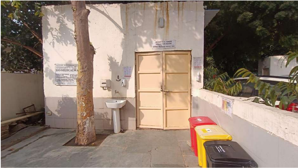
Photograph :- Bio-Medical Waste Storage Area
