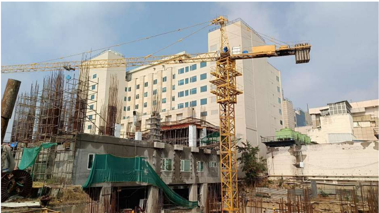
Photograph :- Under-Construction Building
